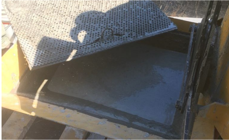
Figure 2.2: Grout consistency prior to installation
