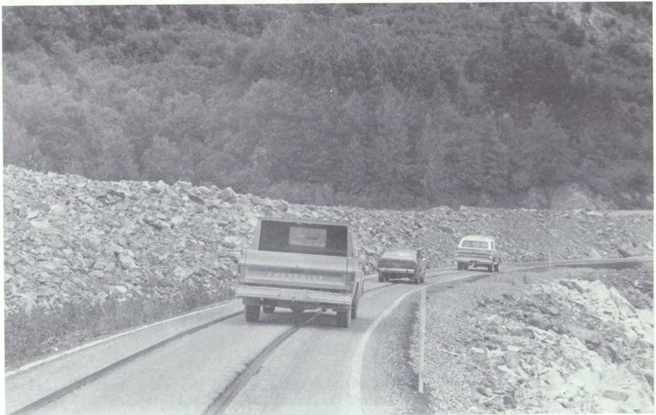
Railbed paving keeps vehicles moving around a major highway reconstruction project on the Seward Highway.
